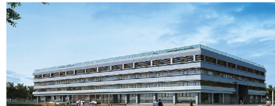
Facility Engineering of Beijing Electric Power Company
